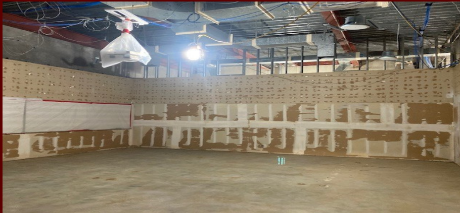
BUILDING K—ROOM 118 PIANO LAB
